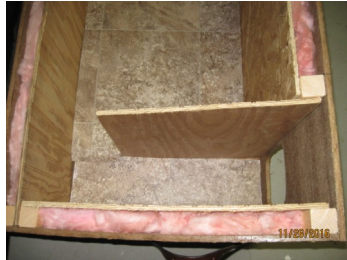
A view of the interior of the Alley Cat winter cat shelter plan displaying double insulated walls, insulation under vinyl flooring and wind guard. Interior will be filled with straw.
